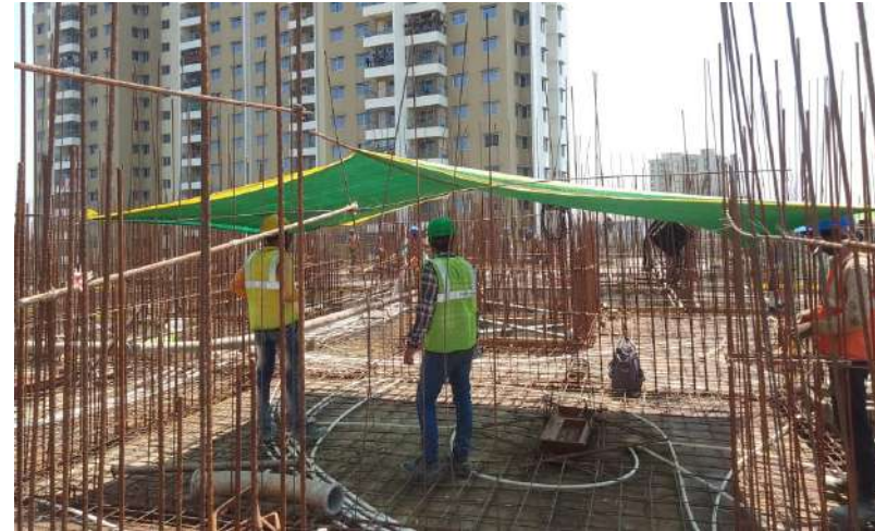
Provision of small shamiana on top working slab
