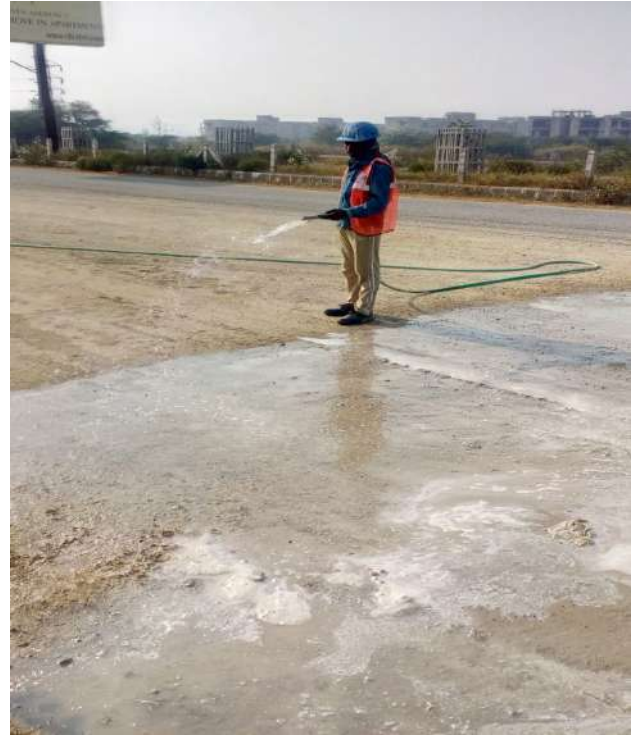
Water Sprinkling at Site for Dust Suppression
