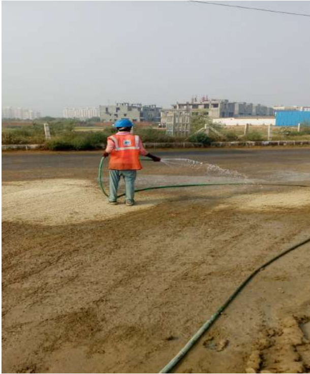
Water Sprinkling at Site for Dust Suppression
