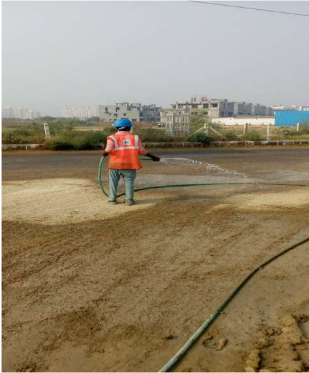
Water Sprinkling at Site for Dust Suppression
