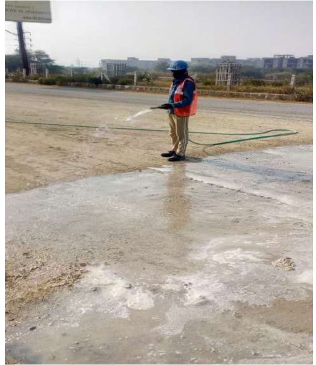
Water Sprinkling at Site for Dust Suppression
