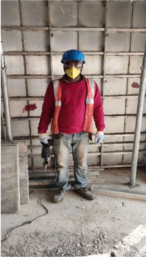
Respiratory Protective Equipment Provided to Worker
