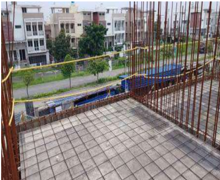
Double layer lifeline rope provided
