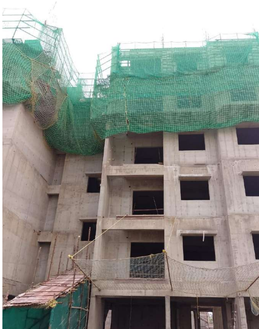
Vertical & Horizontal Net Fixing
