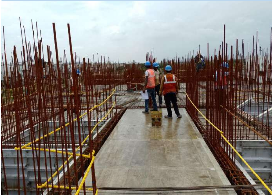
Double layer lifeline rope provided
