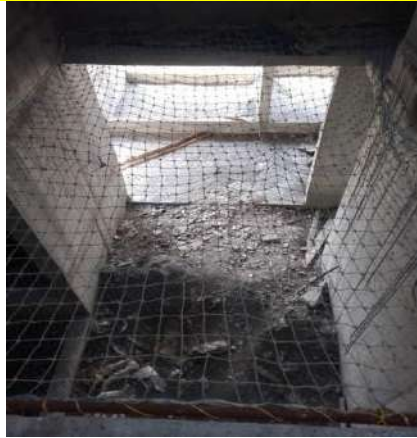
Catch net fixing at OTS and lift shaft area
