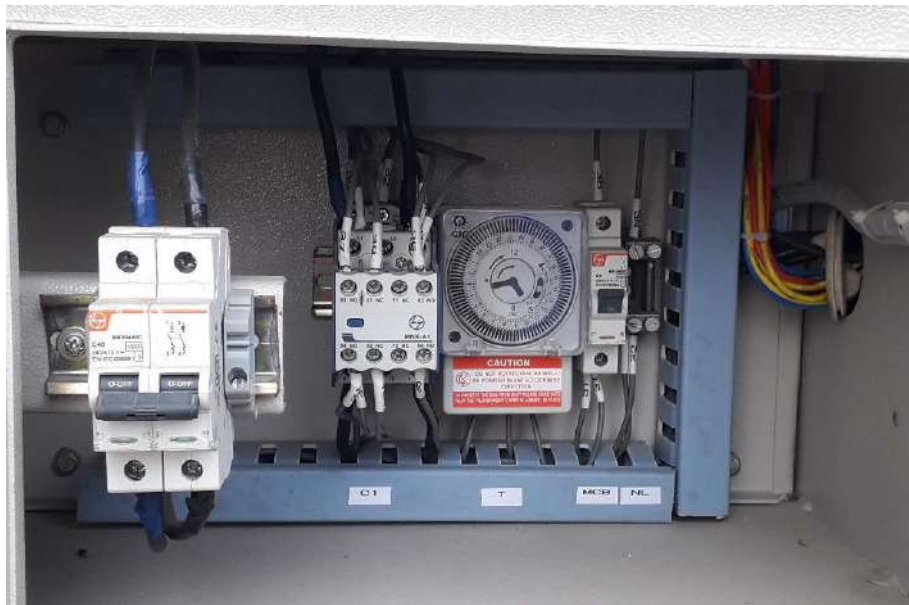
Timer installed in electrical panel
